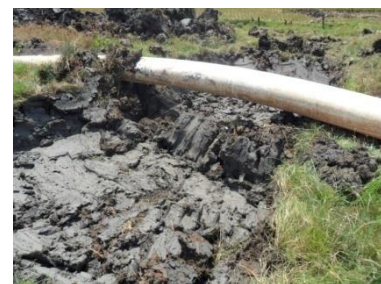
Gambar 1.1 Upheaval Buckling Pipeline
