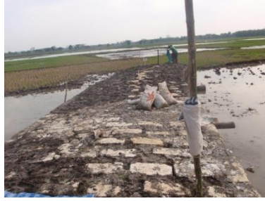
Gambar 1.2 Mitigasi Upheaval Buckling
